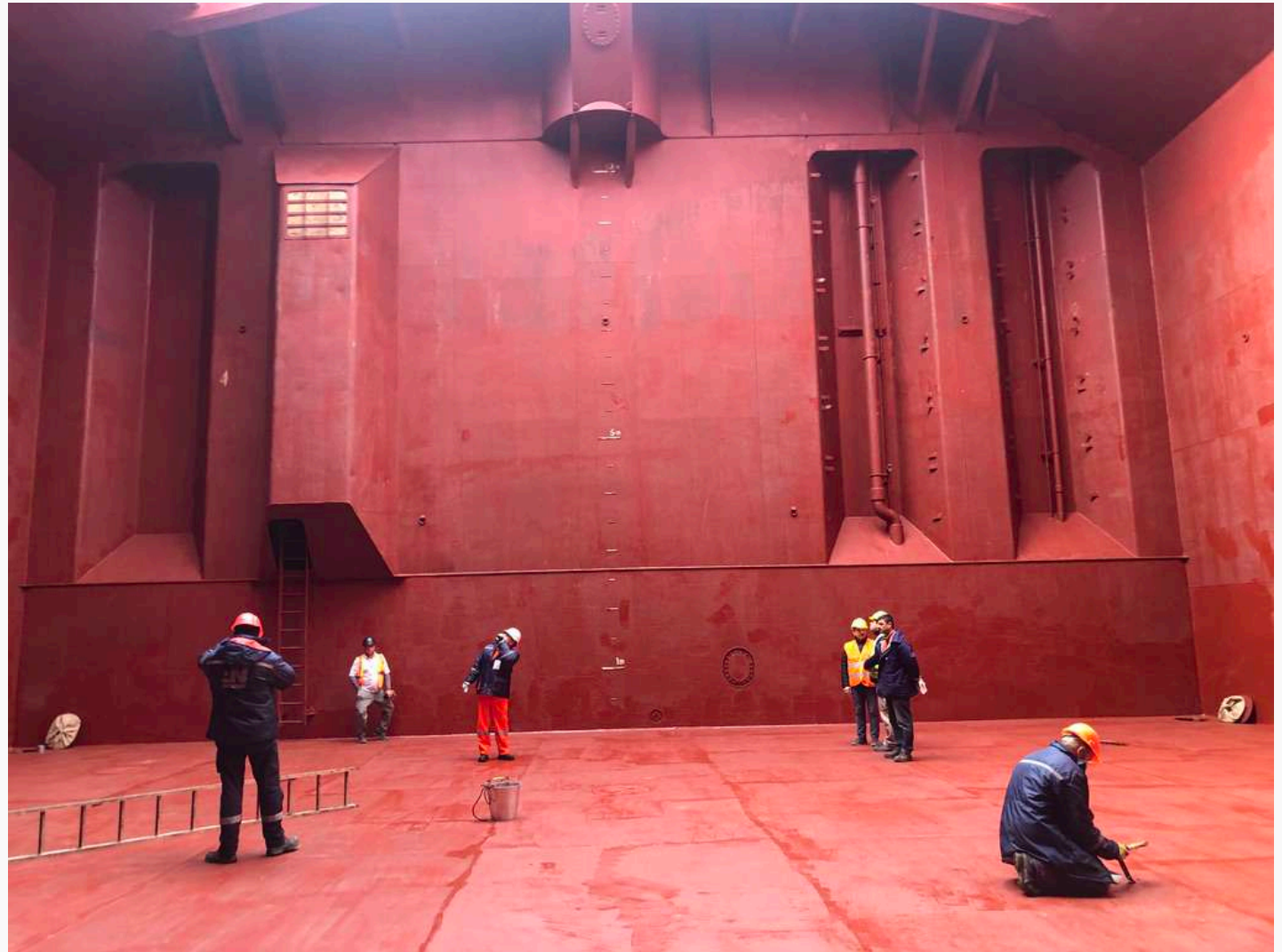
Sweeping and collecting fallen paint
