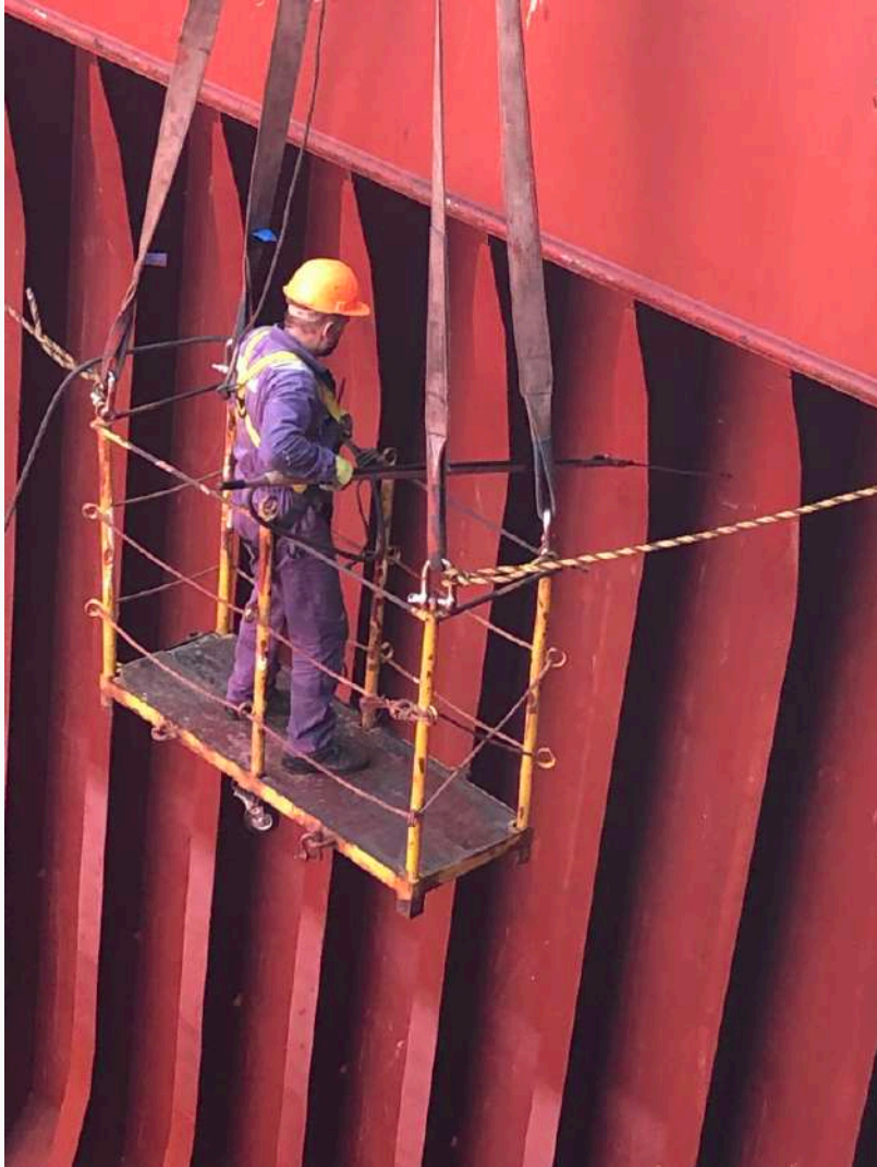
Removing flaking paint with air wand
